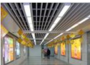
Metro Lighting Project
